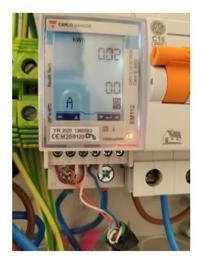
Body + meter: shows correct cabling
